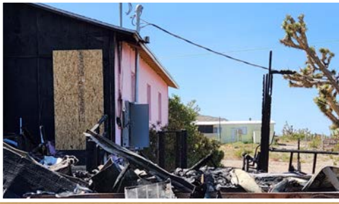
Dolan Springs, AZ Church fire. Renovation Project Fall 2023
