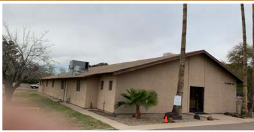
Glendale, AZ Church Fellowship Hall re-roof Project
